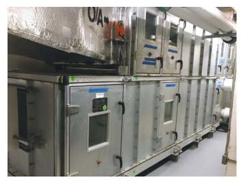
The SA Series Energy Recovery Core Array unit is installed inside of this air handler at NCH.
